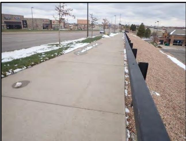
Figure 51: Concrete flatwork in excellent condition over retaining wall
