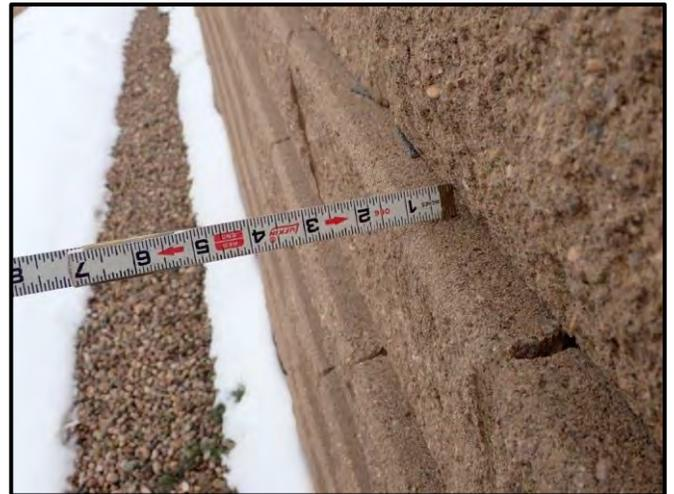
Figure 36: Proper batter of Wall B
