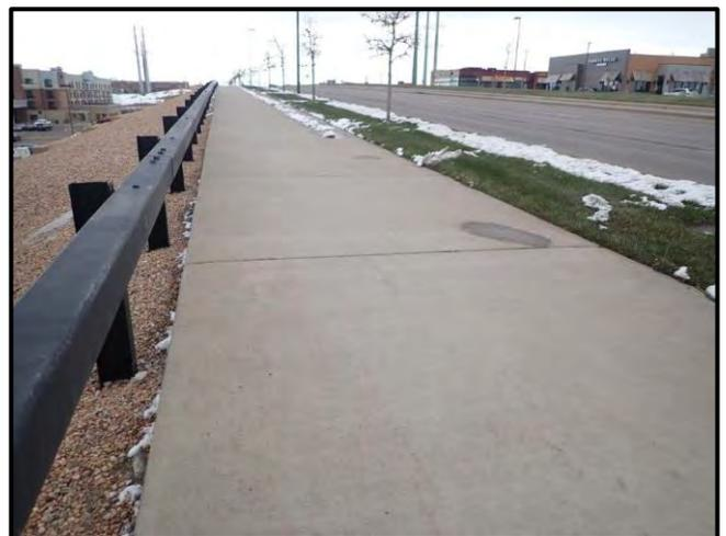
Figure 52: No signs of distress in concrete flatwork over retaining wall
