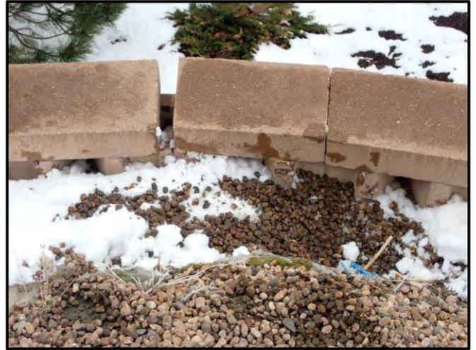
Figure 27: Closeup of soil subsidence behind CMU fascia wall and separation of capstone
