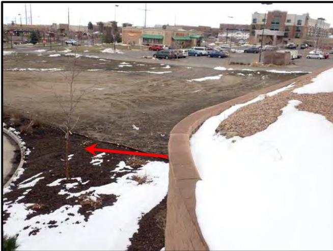
Figure 37: Outside radius of Wall A leans outward approximately  $0.5^\circ$
