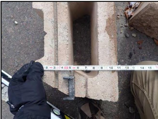
Figure 20: Typical section of CMU with plastic clips still installed
