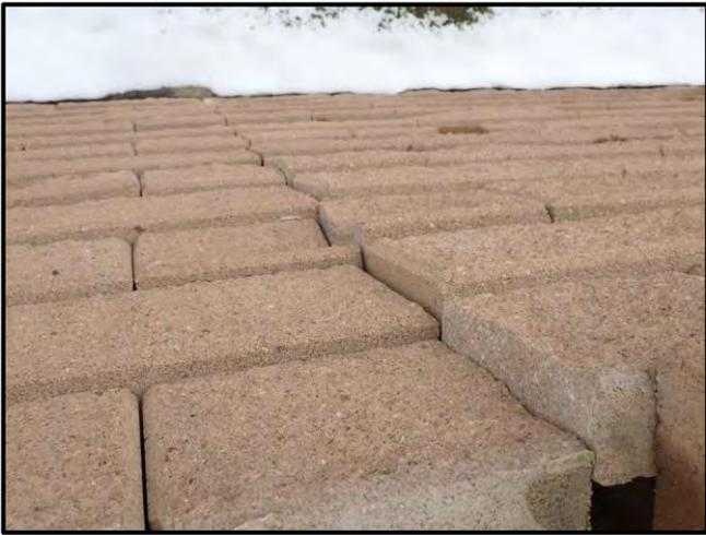
Figure 47: Second view of displaced CMU fascia wall showing the displacement is greater at the top
