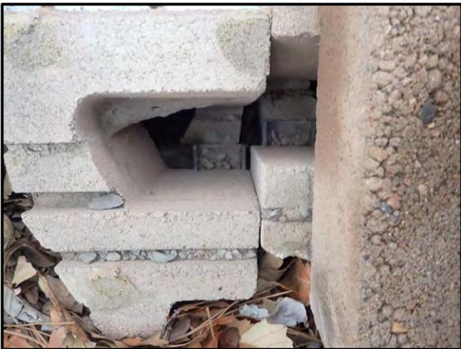
Figure 49: No gravel infill within block void
