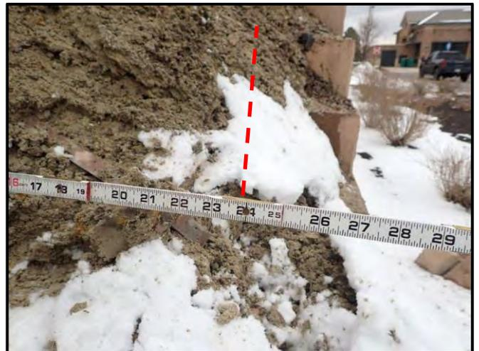
Figure 31: Lateral view attempting to align interior face of CMU fascia wall with folding ruler
