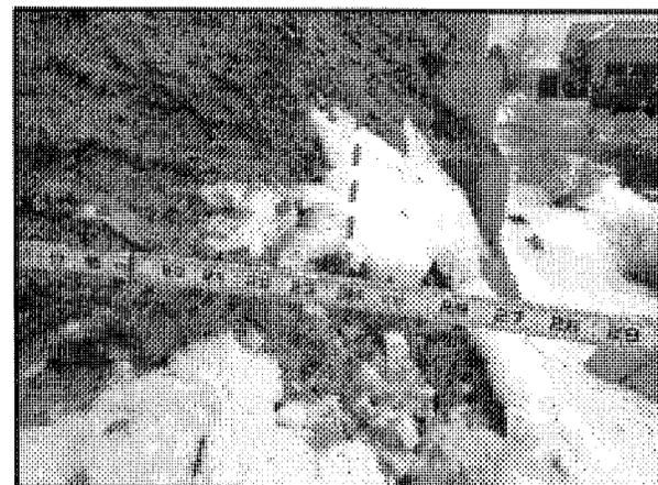
Figure 31: Lateral view attempting to align interior face of CMU fascia wall with folding rule
