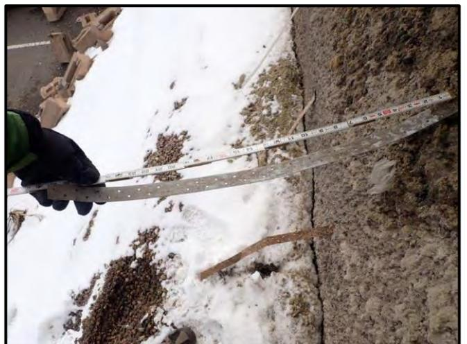
Figure 15: Straight wall tie with no evidence of bend from being turned down into the void of the CMUs
