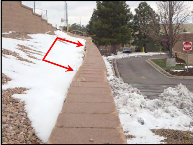
Figure 33: Undulations in Wall A where wall leans outward
