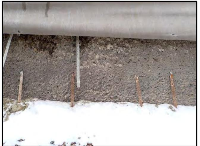
Figure 13: Several wall ties still connected to the shotcrete wall exhibit corrosion
