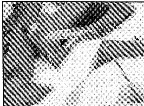
Figure 19: Sharp bend in wall tie where it was bent downward within void of CMU
