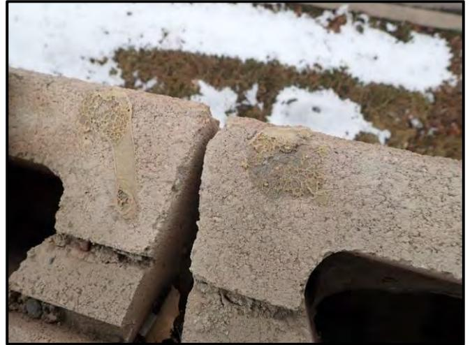
Figure 40: Adhesive on last course of block in Wall A to attach cap unit
