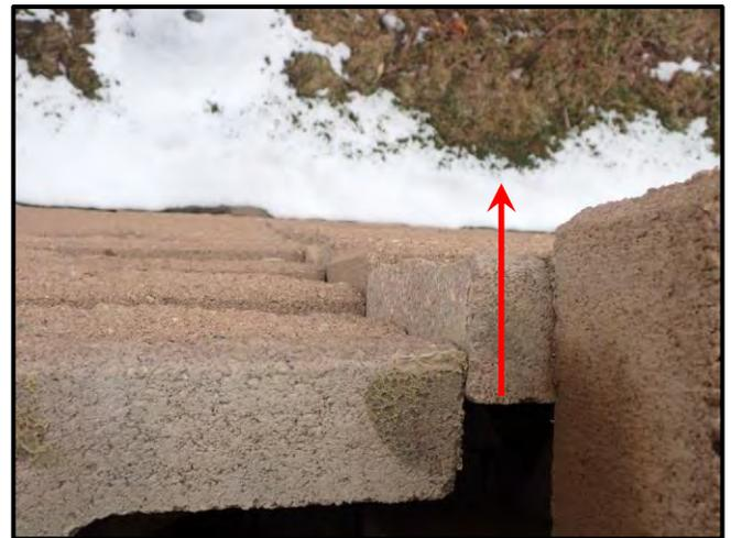
Figure 46: Construction joint showing CMU fascia wall displaced outward
