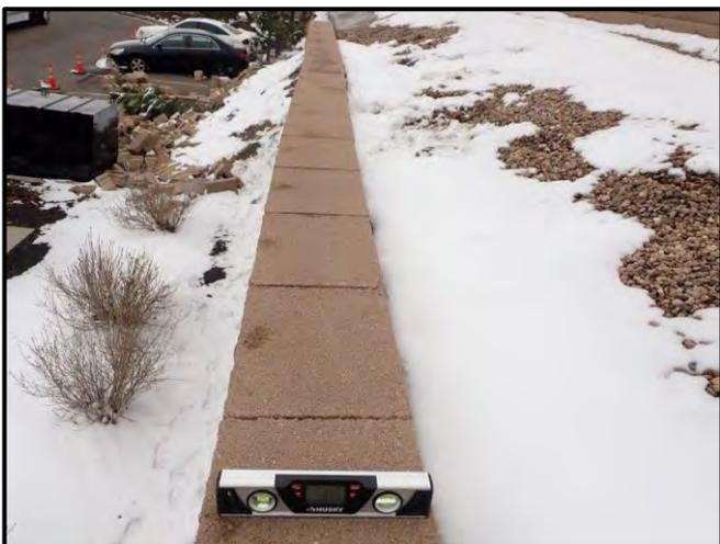
Figure 43: Wall A cap unit leaning outward at 3.9°
