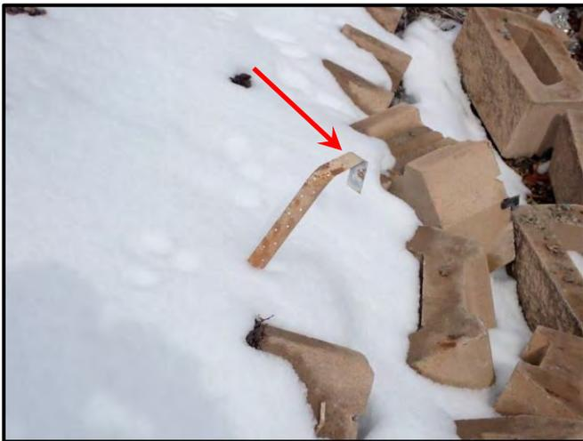
Figure 18: Sharp bend in wall tie where it was bent downward within void of CMU
