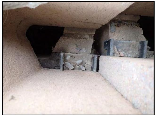
Figure 50: No gravel fill within block void
