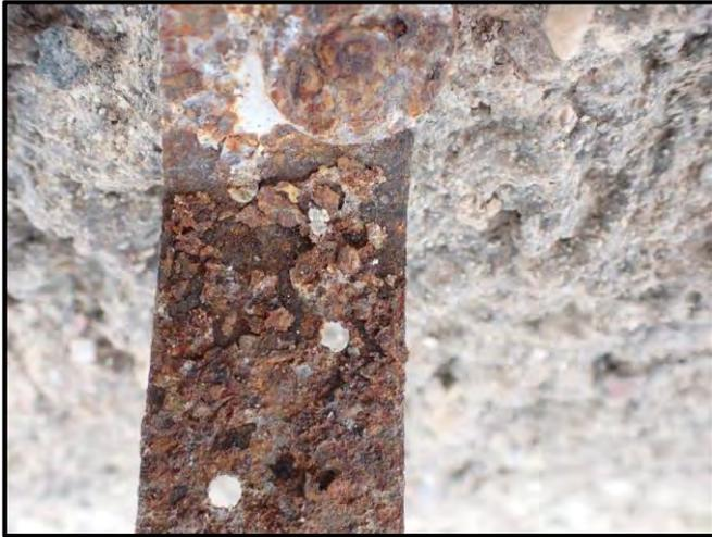
Figure 16: Close up of corroded wall tie
