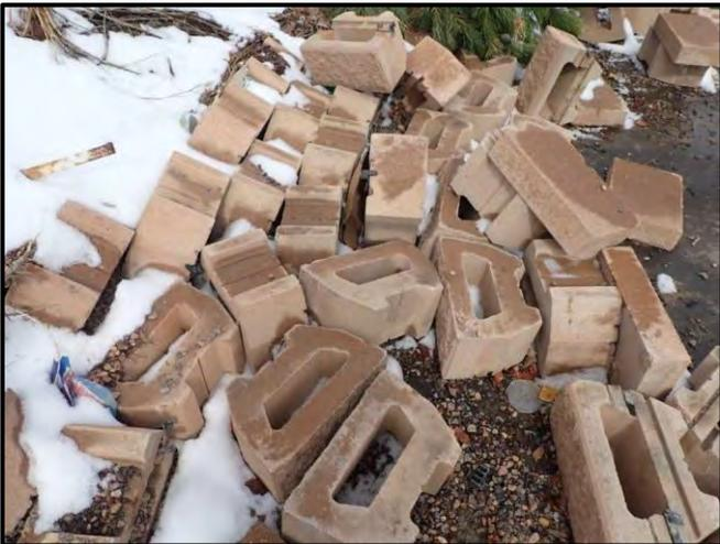
Figure 12: Scattered blocks and gravel fill
