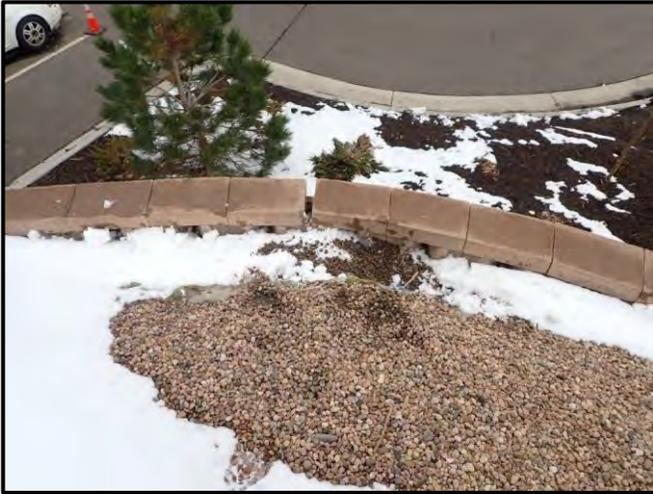
Figure 26: Overview of soil subsidence behind CMU fascia wall with separation between capstones indicating movement
