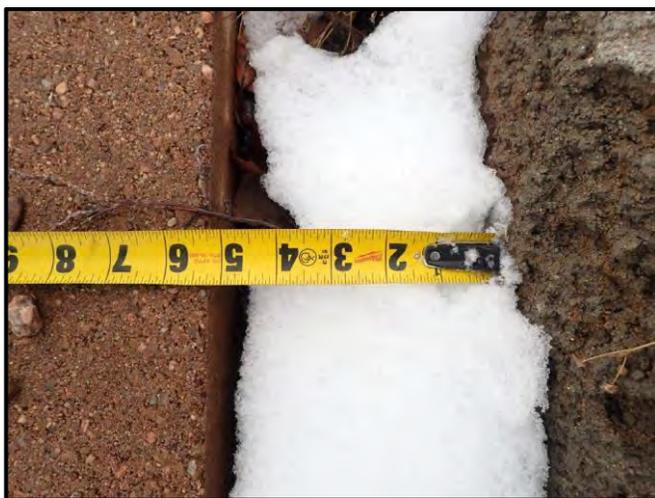
Figure 24: Space between shotcrete wall and back of cap unit approximately 5 inches
