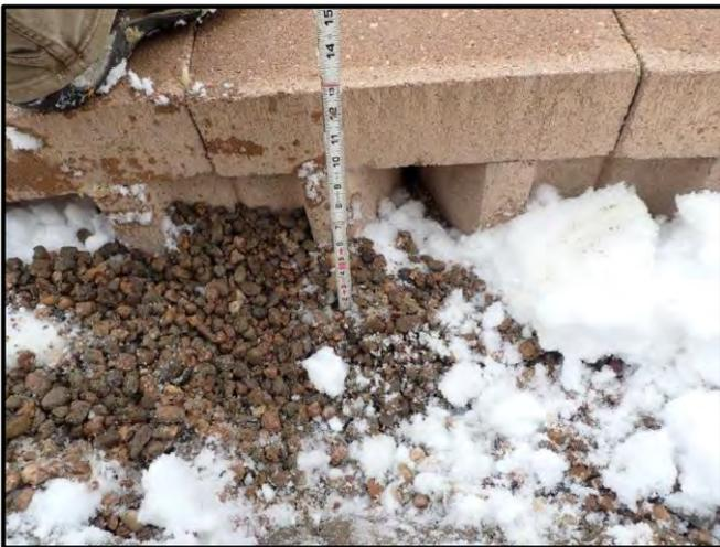
Figure 28: Approximately 12 inches of soil subsidence
