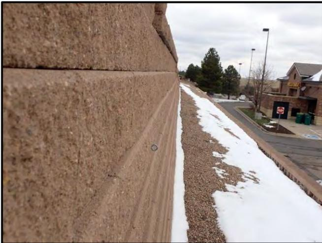
Figure 35: Wall B showing proper batter towards fill
