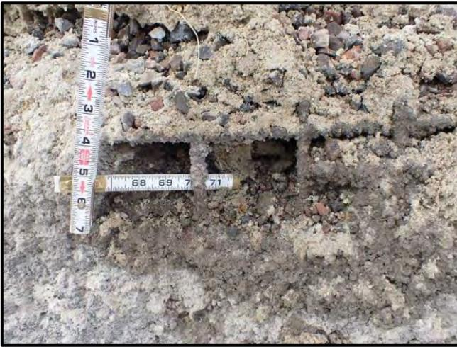
Figure 53: Exposed rebar in shotcrete soil nail wall; designed to have approximately 5 inches of cover
