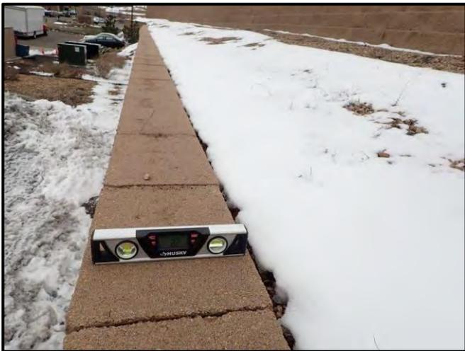
Figure 41: Wall A cap unit leaning outward at 2.2°
