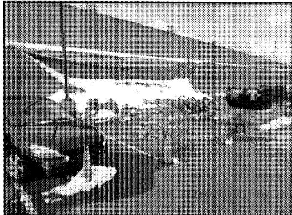
Figure 11: Overview of localized collapse of retaining wall
