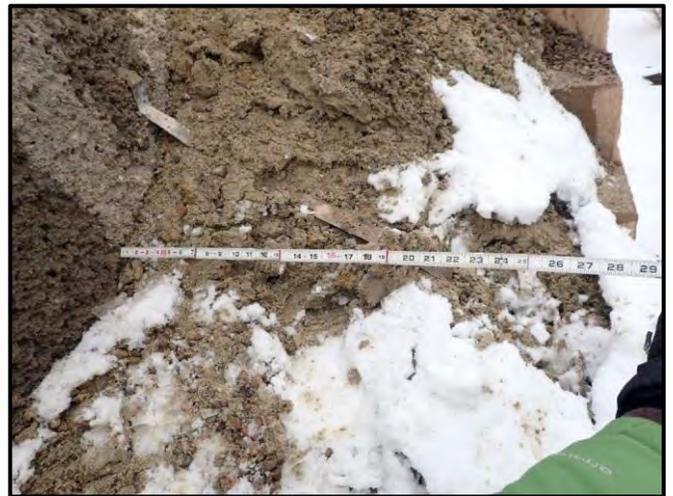
Figure 29: Collapsed area showed approximately 24 inches of backfilled space between walls
