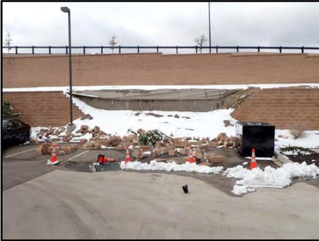
Figure 10: Overview of localized collapse of retaining wall
