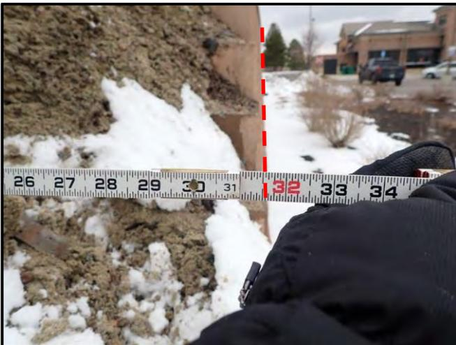
Figure 30: Lateral view attempting to align exterior face of CMU fascia wall with folding ruler
