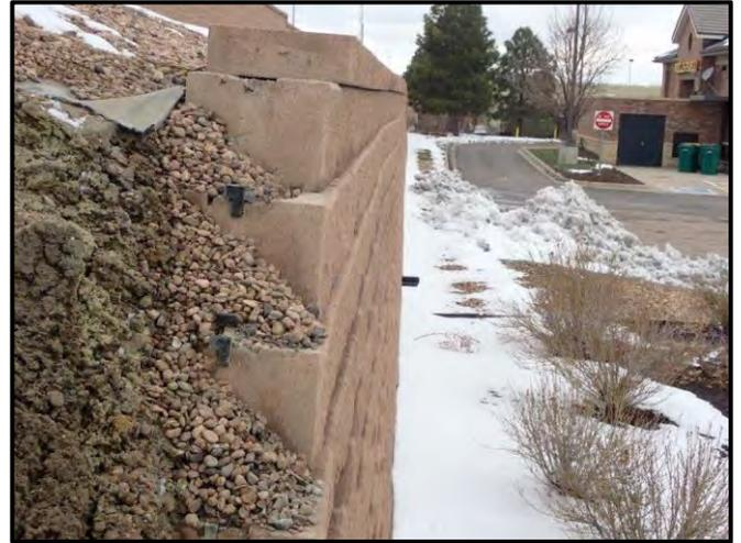
Figure 34: Undulations in Wall A where wall leans outward
