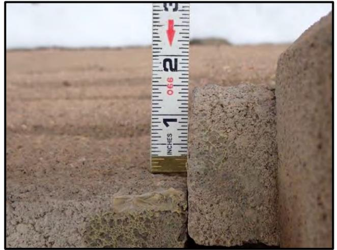
Figure 48: Displaced CMU fascia wall approximately 1.5 inches outward
