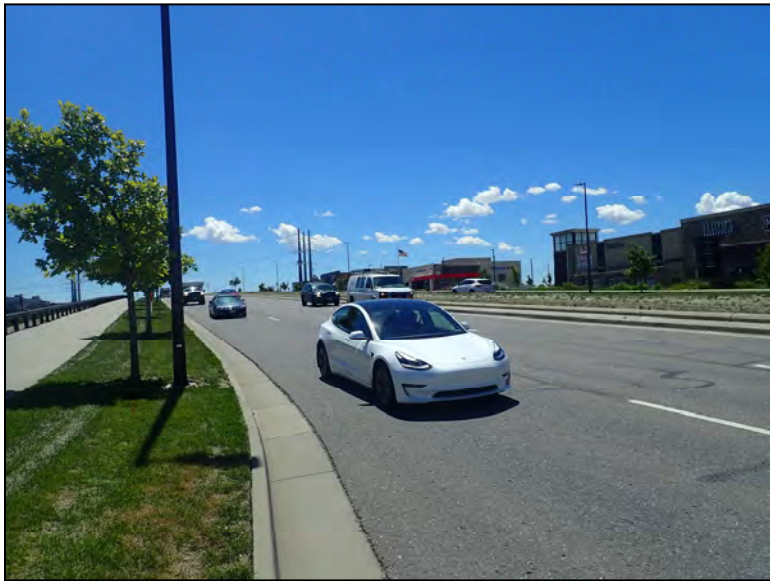
Roadway Carried, Looking Southeast
