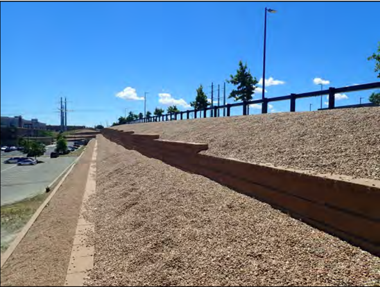
Elevation, Looking Southeast
