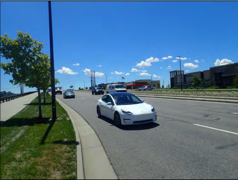
Roadway Carried, Looking Southeast
