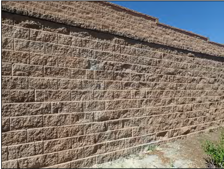
View of Repaired Area in Wall Facing at Sta. 7+28
