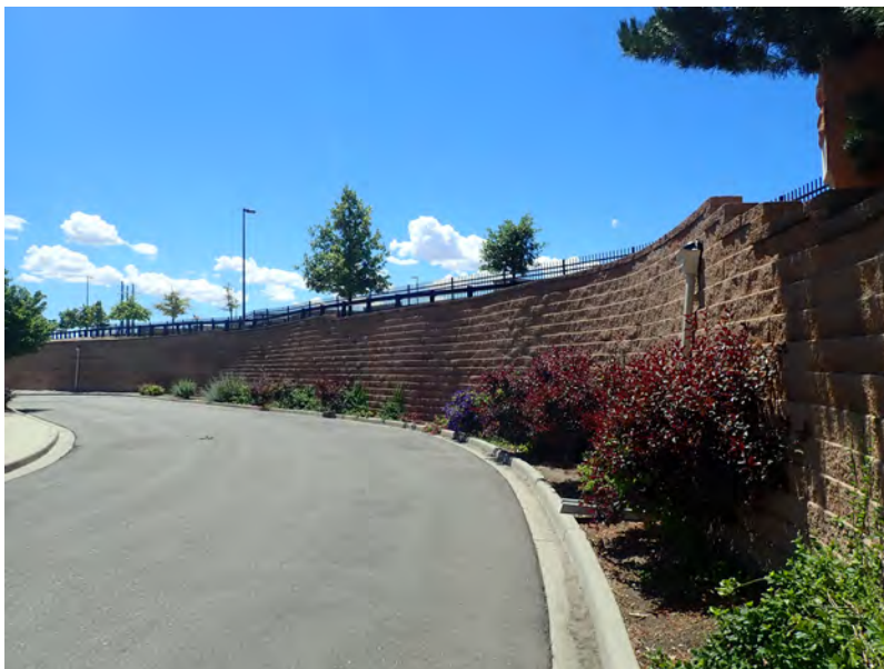
Elevation looking southeast
