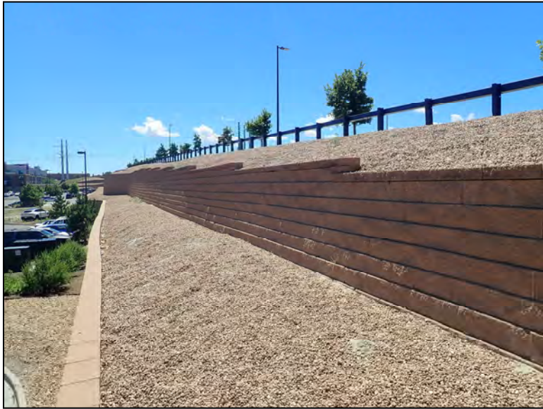
Elevation, Looking Southeast
