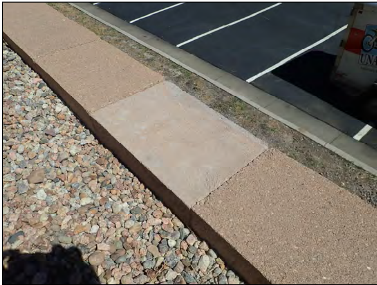
Typical Replaced Masonry Capstone at Top of Wall
