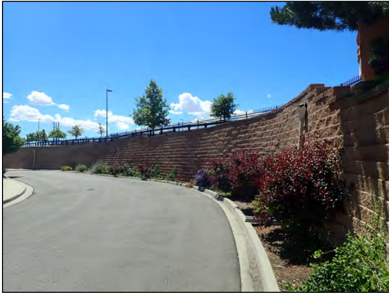
Elevation, Looking Southeast
