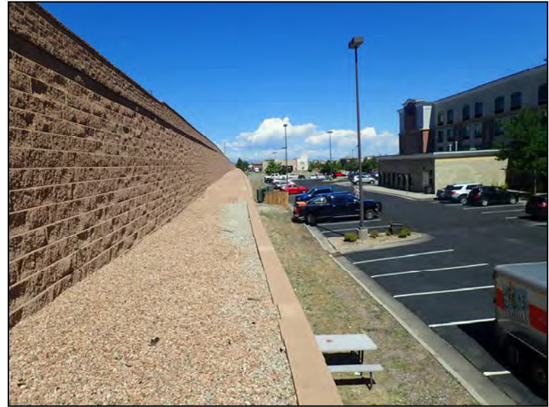
Areas of Newer/Replaced Gravel Ballast at Top of Wall at Sta. 14+55
