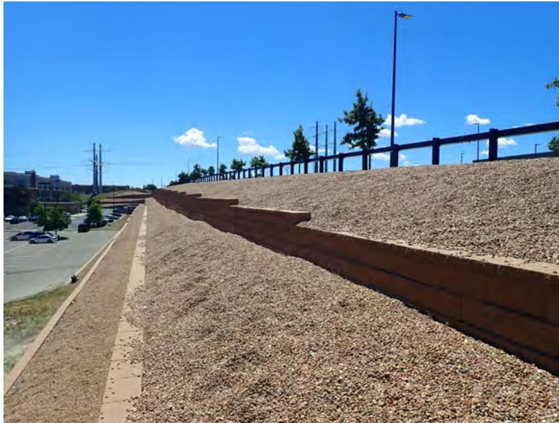
Elevation looking southeast
