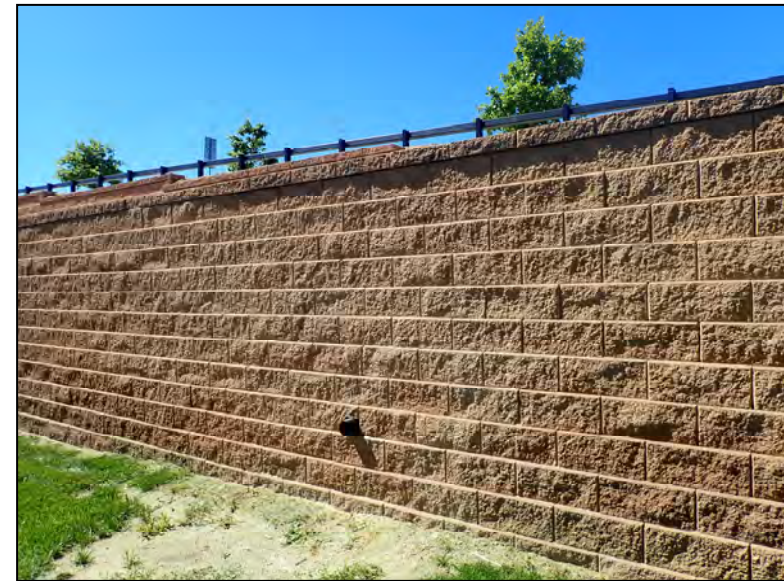
View of Repaired Area in Wall Facing at Sta. 5+55
