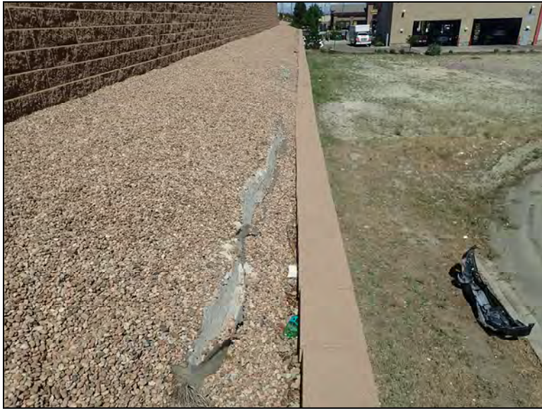
Typical Exposed Shotcrete Wall Behind Top of Masonry Wall Facing
