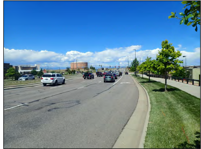
Roadway Carried, Looking West
