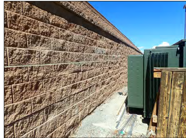
View of Repaired Area in Wall Facing at Sta. 14+55
