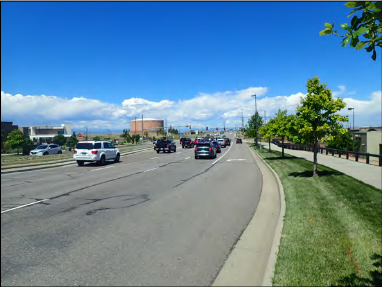
Roadway Carried, Looking West
