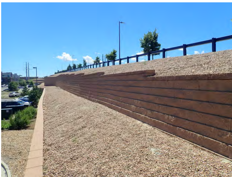
Elevation looking southeast
